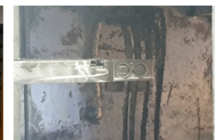
(b) Installation of manifold
