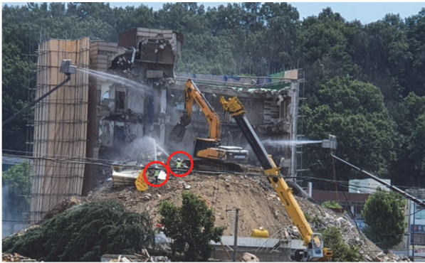
(a) Manual water spraying in a demolition site [5] (Adapted from Ref. 5 on the basis of webpage)
